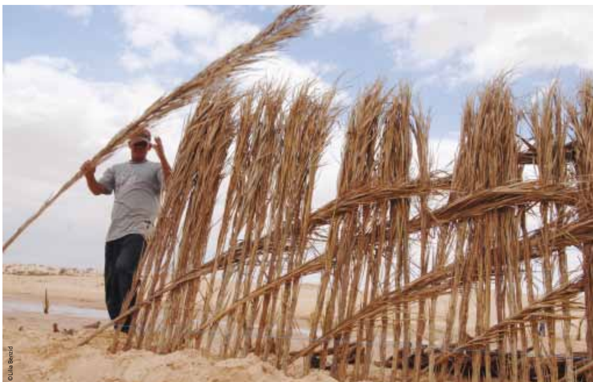
Consolidating the dunes, Noueil - Tunisia
