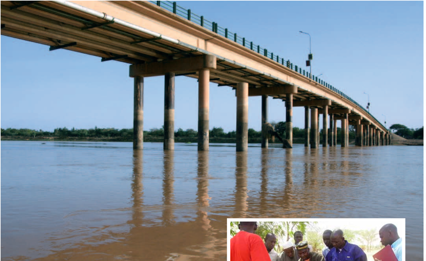
Bridge across the Niger River – Niamey, 2009
