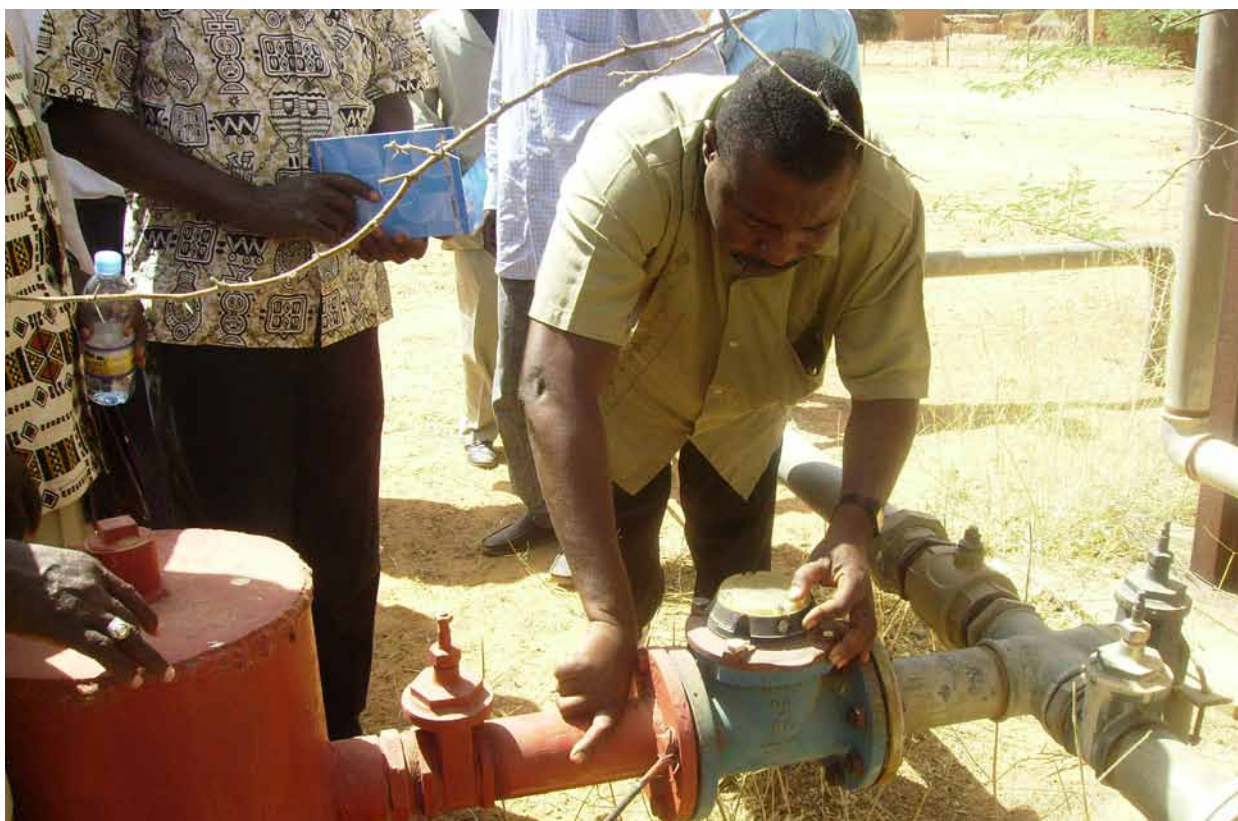
Hydraulic installation, Banizoumbou – Niger, 2007
