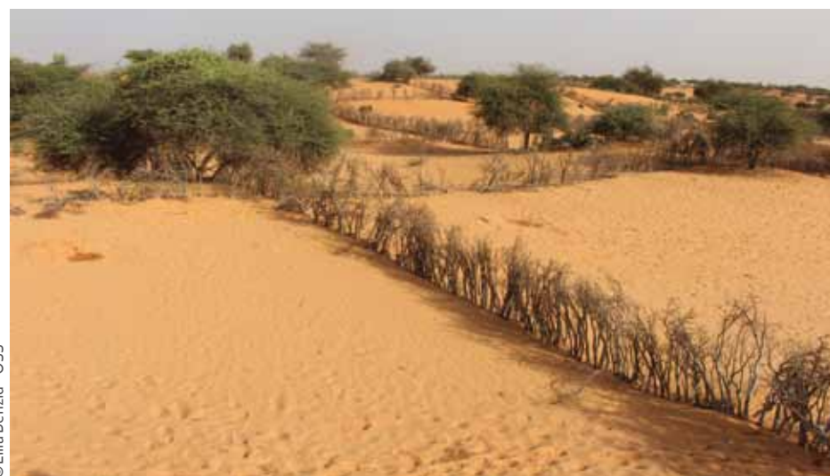
Sand dune stabilisation works, Rosso, Mauritania
